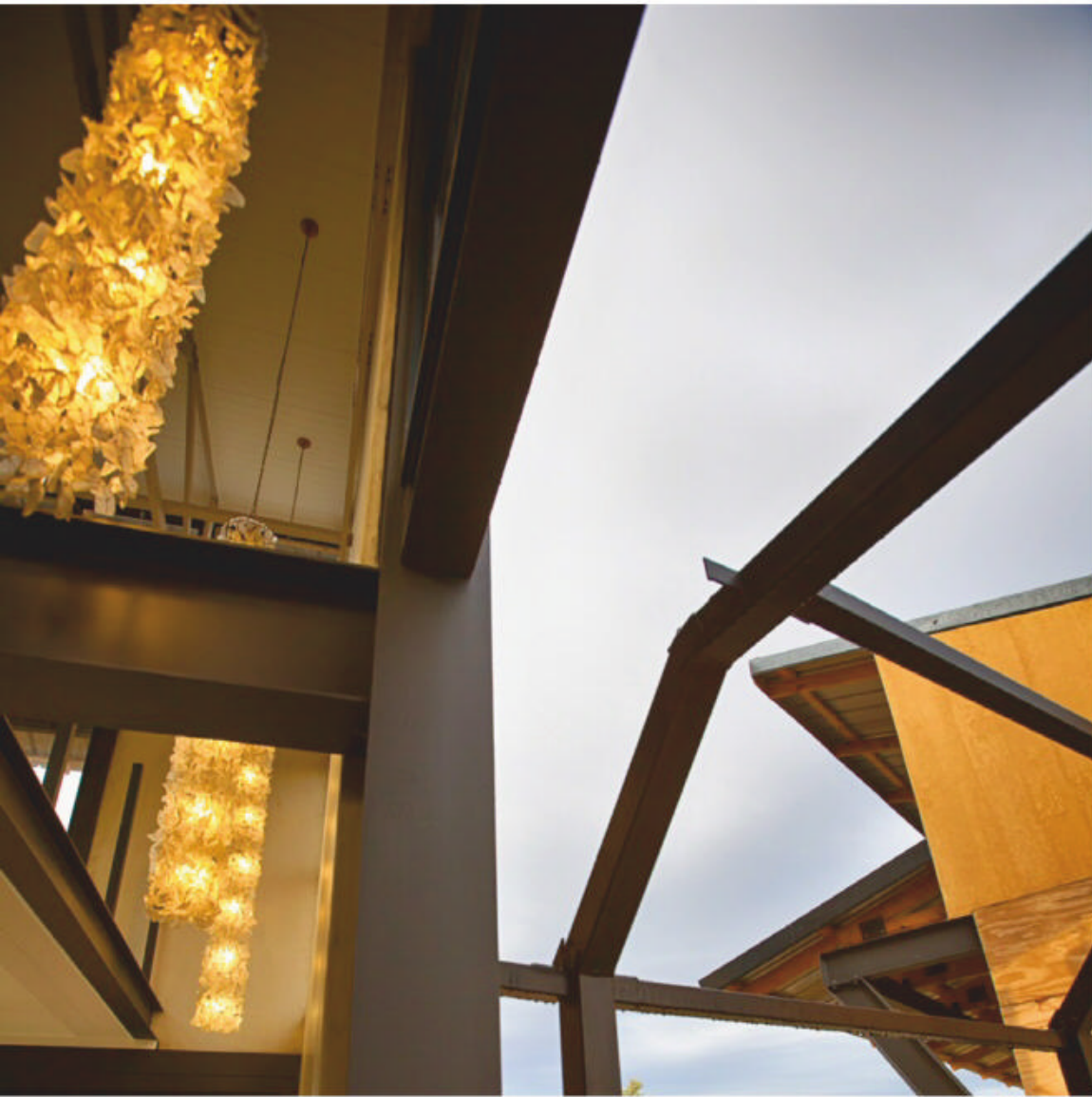
Installation of drop-down light fittings made from reclaimed glass bottle pieces and wires and using LED lights.
