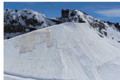
Fleece to prevent ice loss on the access ramp.
